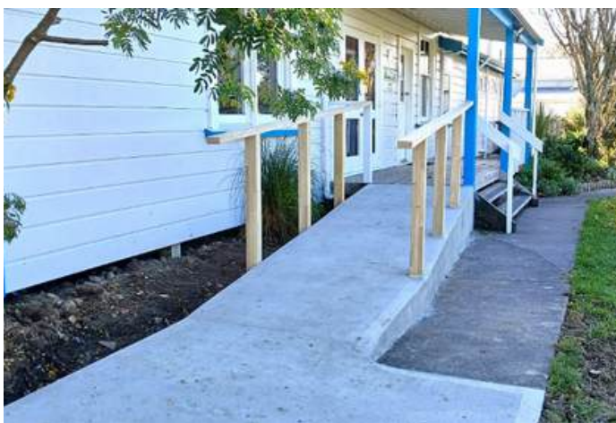
Above: Newly built ramp by our support office.
